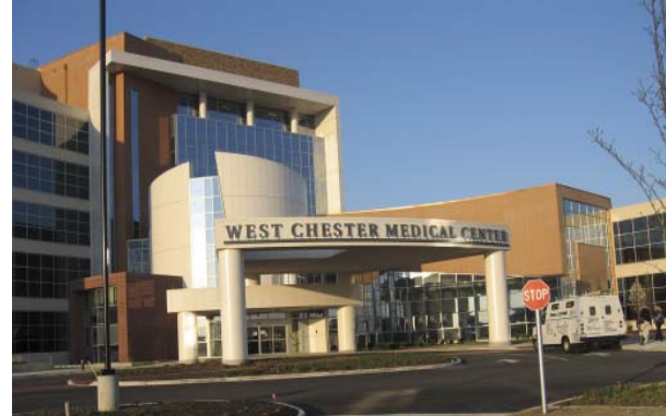
The new West Chester Medical Center - West Chester, OH
